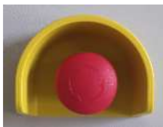
Fig. 4-3 EMERGENCY STOP switch to interrupt MV mains supply
